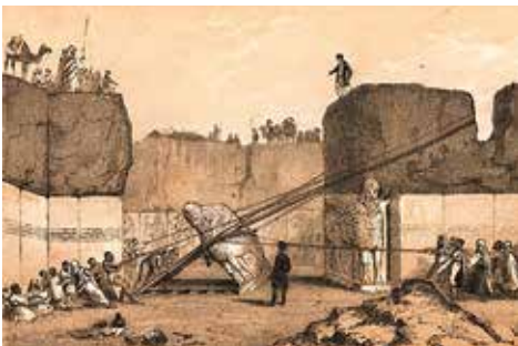
Excavation of Nineveh
